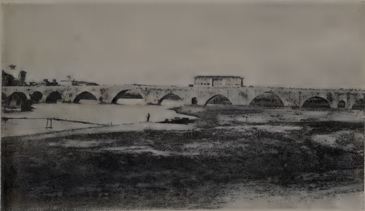
FIG. 11.—The Bridge over the Saros at Adana (Mrs. Christie of Tarsus). To face p. 176. See p. 274.
